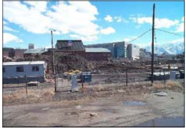
500 West Park Blocks Existing Conditions
